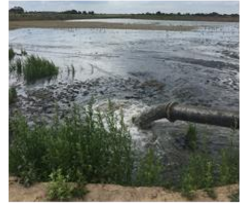
This is a lagoon similar to those that have been constructed so the dredged material can settle – the water will run into nearby drains and silt eventually be mixed into the land.
