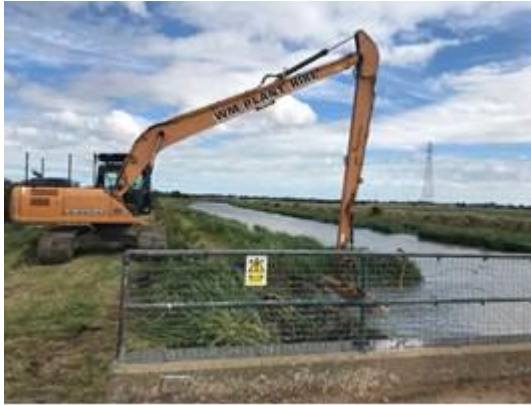
Weed cutting was completed mid September to get the roots out of the middle of the river ready for dredging.
